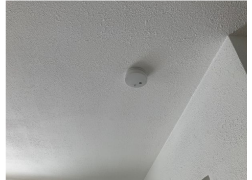
2nd Floor Back Bedroom
