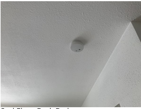
2nd Floor Back Bedroom
